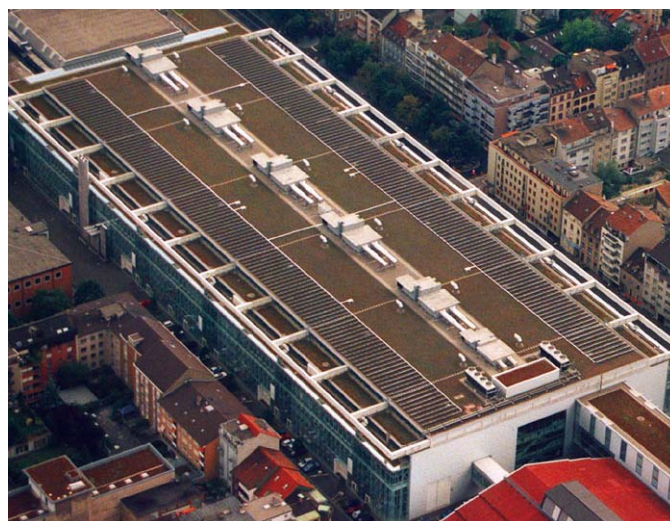
Fig. 4 - 240 kWp PV system on the Basel fair building. (photo energiebüro)
