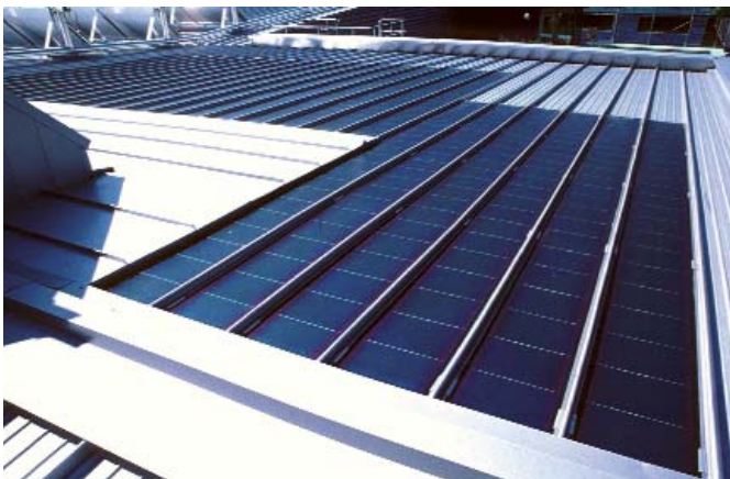
Fig. 1 - Photovoltaic metal roof system using amorphous thin film solar cells. (photo NET)
