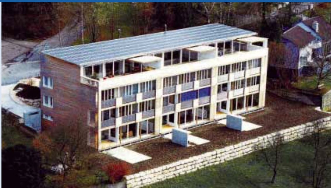
Fig. 2 - Sunny Woods: 6 kWp amorphous silicon system in an energy optimised multifamily house in Zurich.
