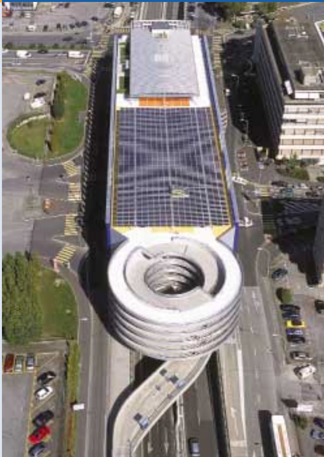
Fig. 3 - Parking de l'Etoile: 143 kWp on the roof of a parking house in Geneva.
