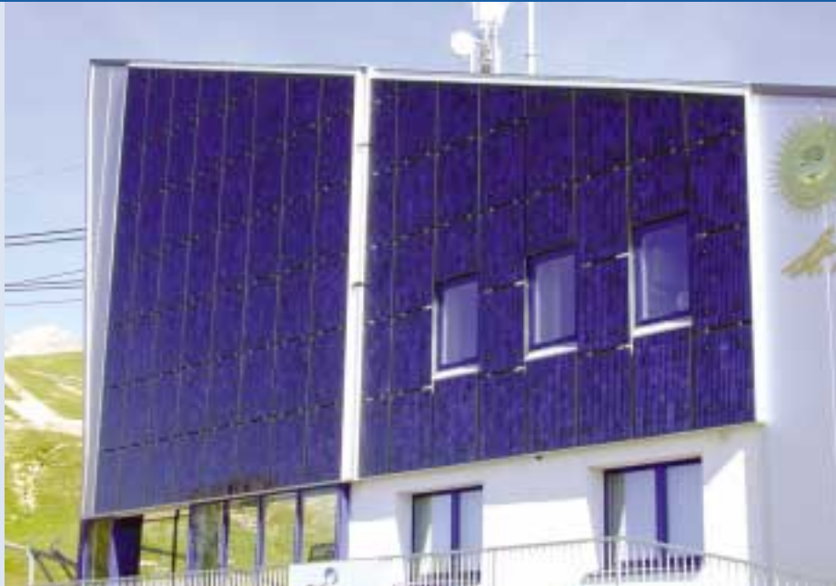
Fig. 3 - 9,7 kWp façade system at the cable-car station Piz Nair in St. Moritz. (photo: NET)
