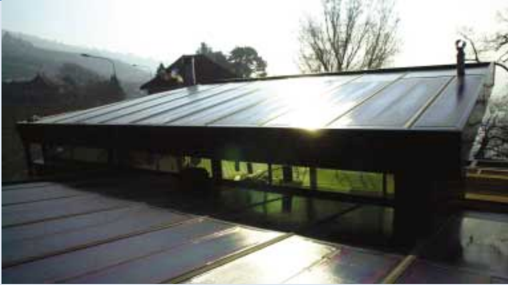
Fig. 1 - 5,5 kWp Freestyle® thin film system on the roof of a single-family house in Lutry. (photo: Solstis)
