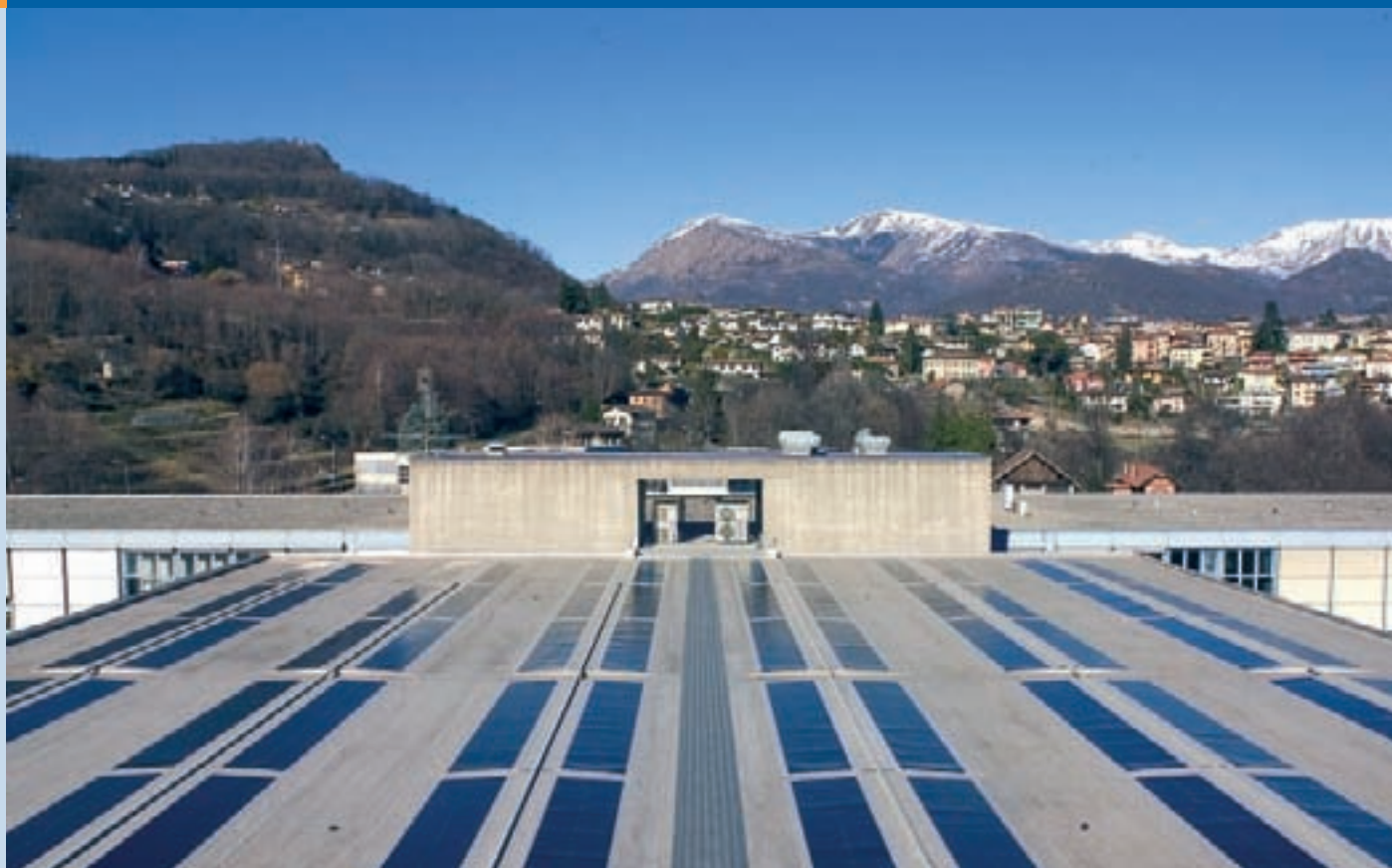
Fig. 2 - 15,4 kWp flat roof PV system using the Sarnasol product (photo Sarnafil).
