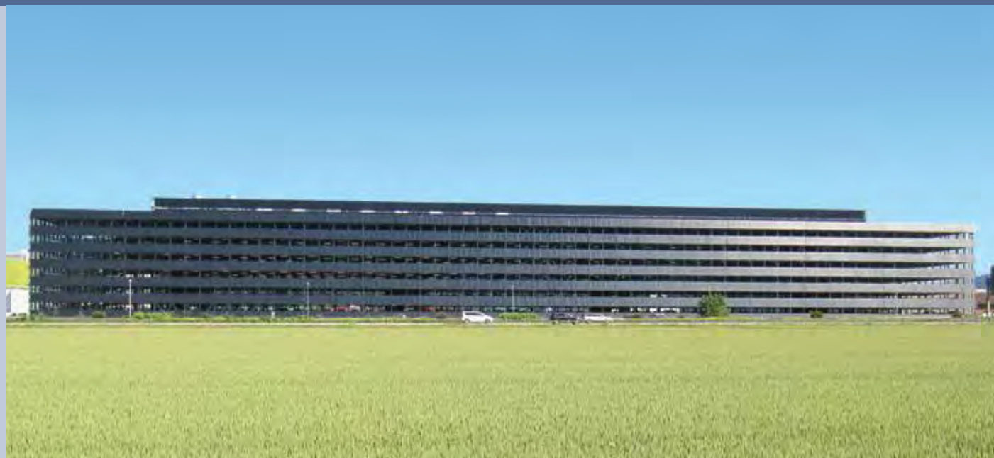
Fig. 1 – Swissolar Prize Winner 2017: The most powerful PV façade in Switzerland on the F. Hoffmann-La Roche AG's parking garage in Kaiseraugst, Switzerland. This façade system has a total installed capacity of 633 kWp and an estimated production of 473 000 kWh per year (Photo: © BE Netz AG, Ebikon).
