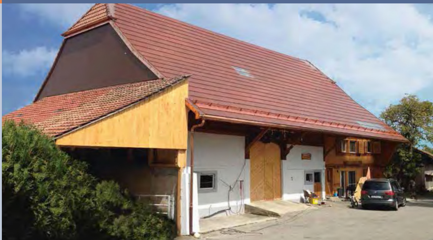
Fig. 2 – A southwest view of the PV installation on a farm house in Ecuwillens, Fribourg, Switzerland. With their terracotta appearance, these innovative PV roof tiles provide a perfect integration into the townscape (photos: © CSEM & © ISSOL).
