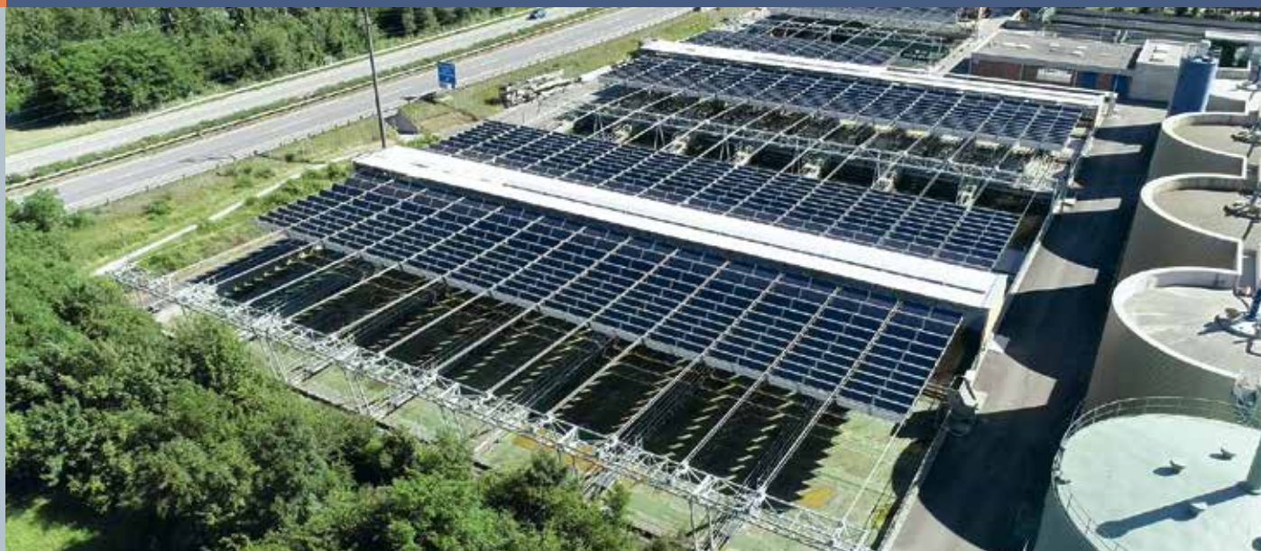
Fig. 5 - dhp has realized the world's first solar folding roof across a sewage infrastructure, a consistent double use of already sealed land for solar power generation in urban infrastructures and with 100% self-consumption. Following a pilot plant with the HORIZON solar folding roof, the system was extended to a capacity of 643 kW in 2018 (Photo: © dhp technology).
